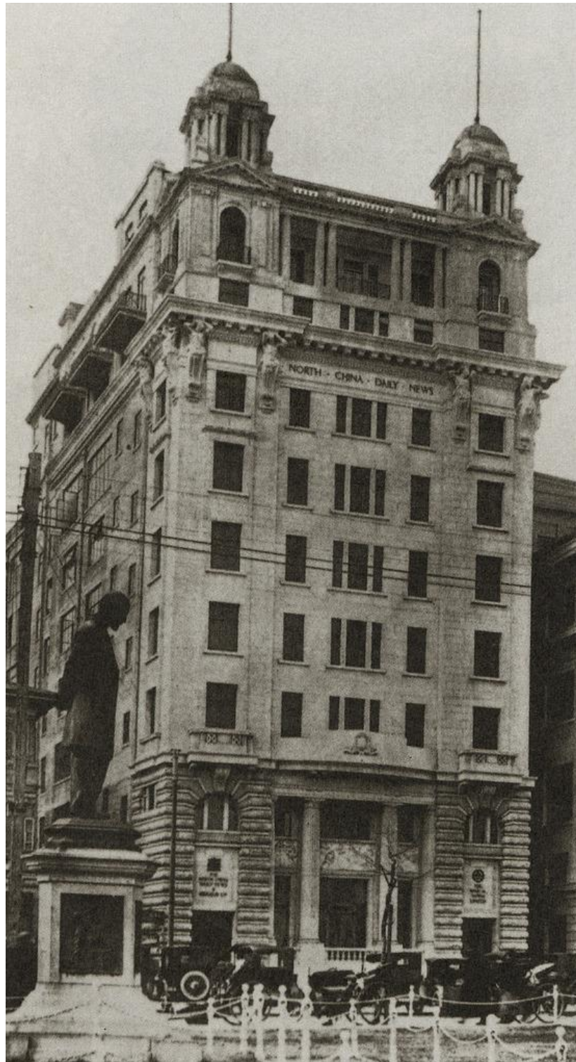
Fig. 1-15 Northern China Daily News Building. Accessed April 2022.
