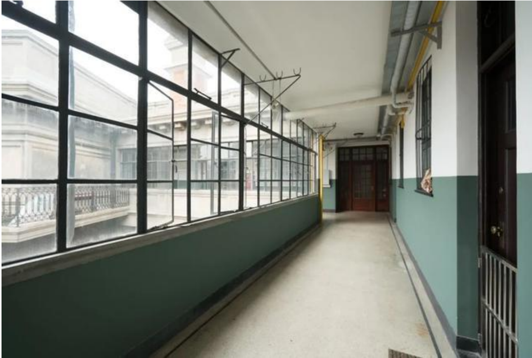
Fig. 1-22: Hallway, renovated and bottom half painted green, 2022. Sina, accessed April 2022, https://finance.sina.com.cn/jjxw/2022-03-23/doc-imcwipii0115012.shtml .
