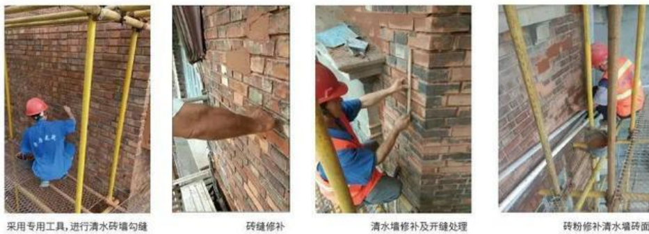
Fig. 3-6: Work in progress for restoring the brick surface.
