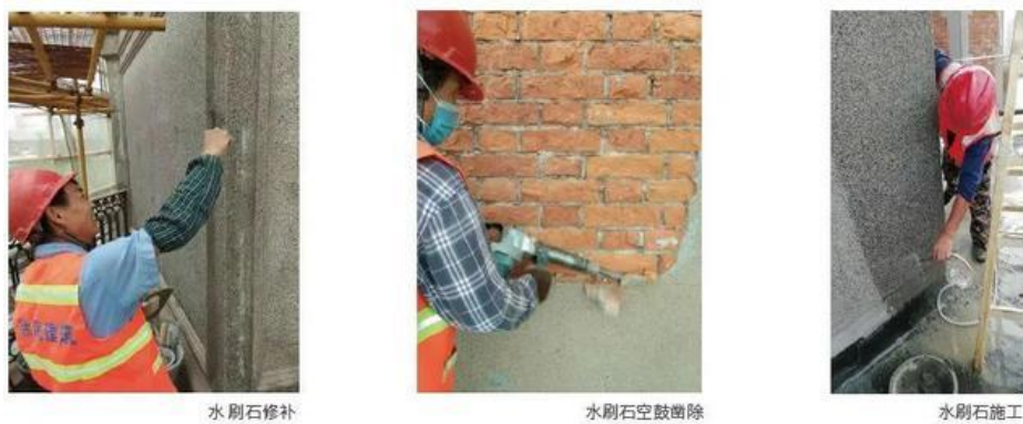
Fig. 3.7: Work in Progress for restoring the stone surface.
