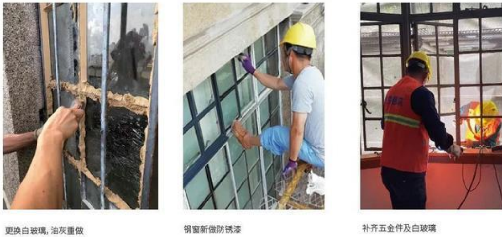
Fig. 3.8: Work in Progress for fixing the windows.
